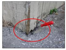
2.1 Item 3(Picture) Siding in contact with grade is vulnerable to water damage
